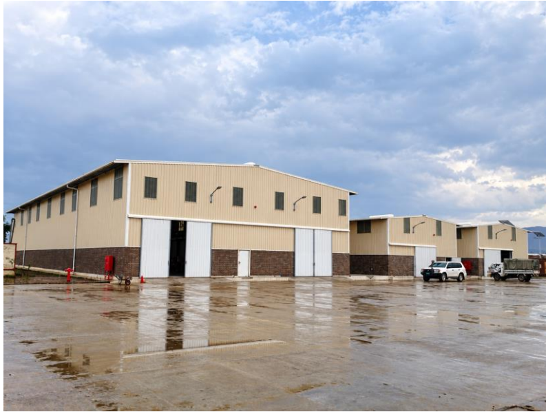
WFP warehouse programme | Completed warehouse blocks and service yard
