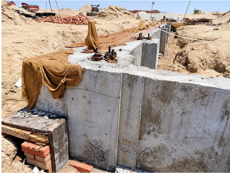
WFP warehouse programme | Concrete foundation line and setting-out activity
