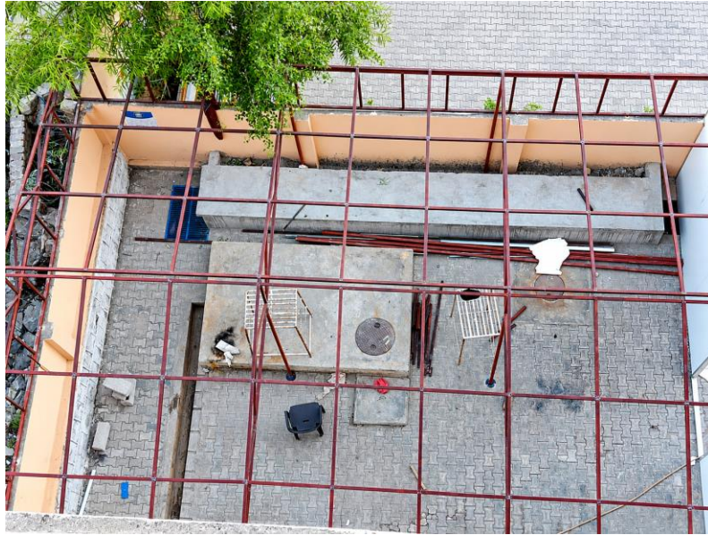
AIMS School and College Islamabad | Overhead structural framework during execution
