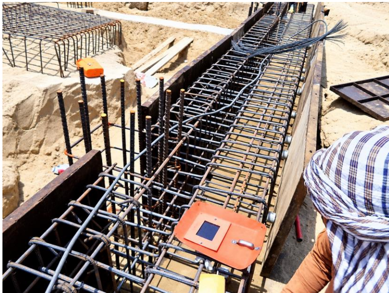
WFP warehouse programme | Reinforcement cage and formwork preparation
