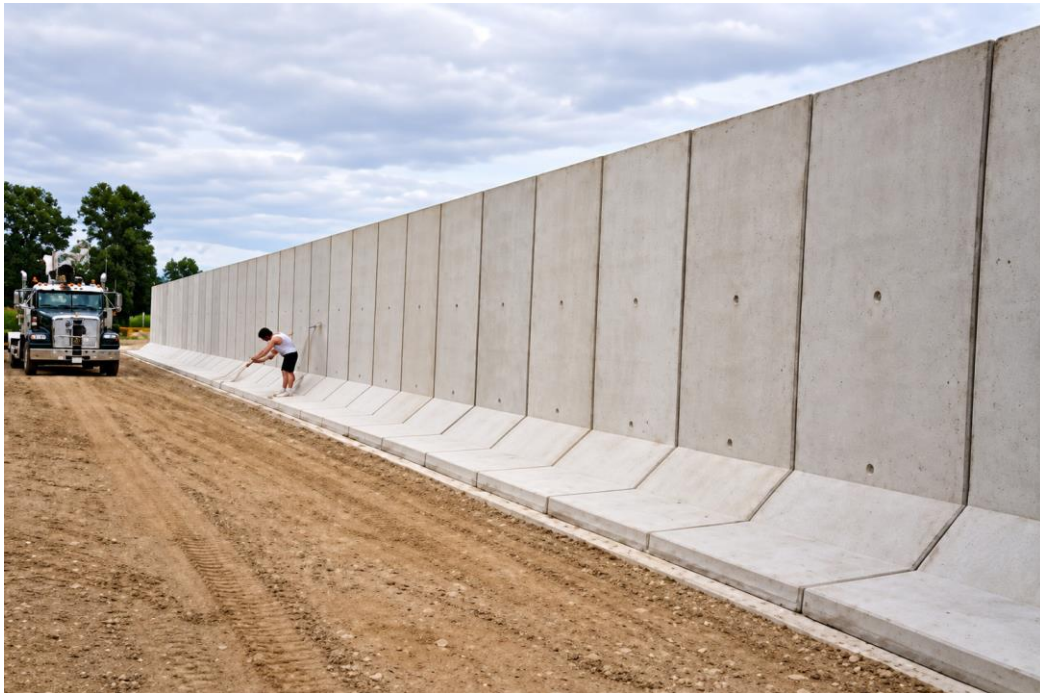
Protective civil works portfolio | Concrete perimeter wall and site approach
