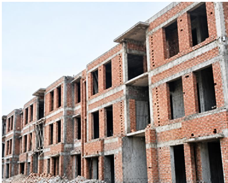
Residential construction portfolio | Multi-storey masonry and concrete construction
