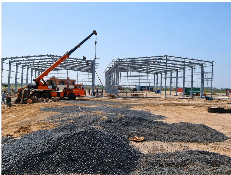
WFP warehouse programme | Crane-assisted steel-frame erection
