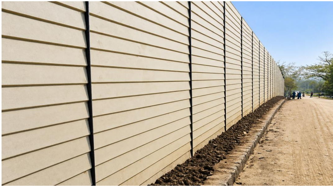
Protective civil works portfolio | Continuous panelled perimeter construction
