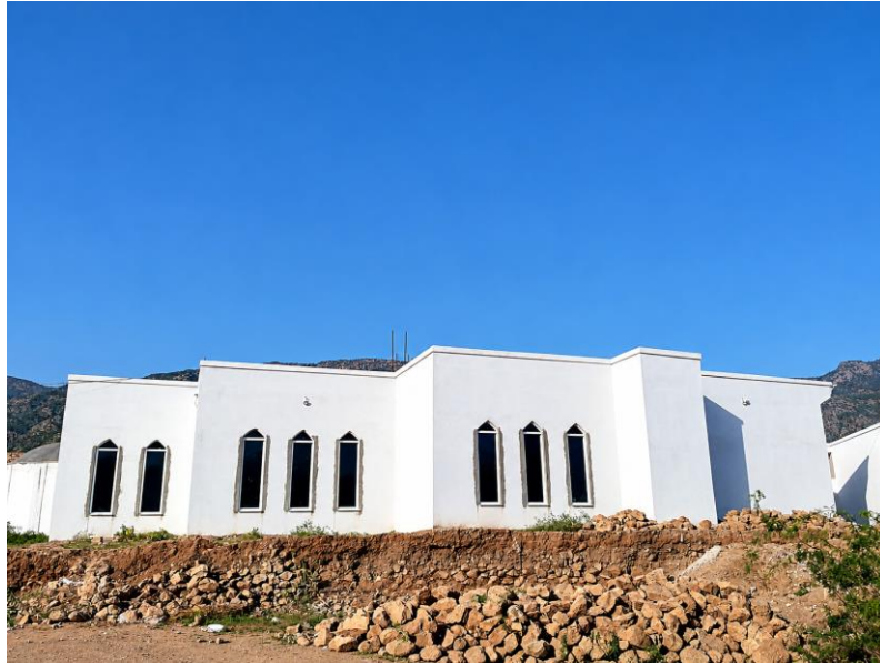
World Federation Alizai Masjid project | Finished exterior envelope
