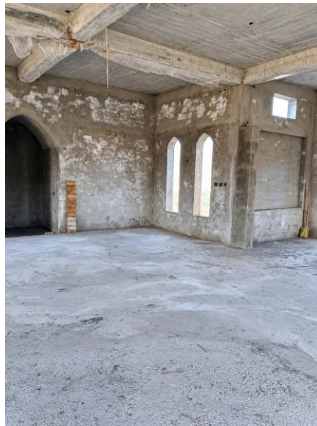
World Federation Alizai Masjid project | Prayer hall at plaster and preparation stage
