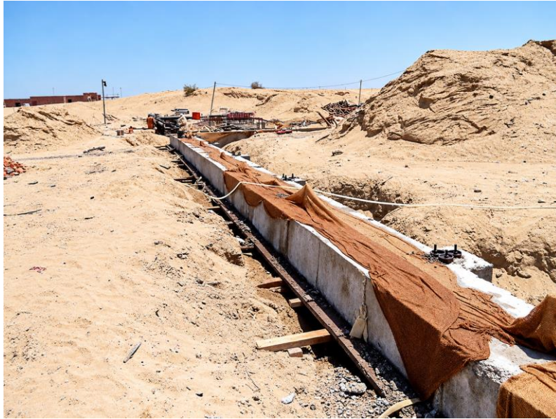
WFP warehouse programme | Long foundation run with protective covering
