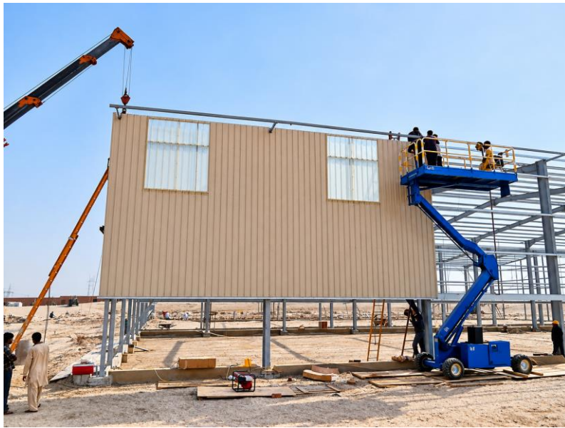
WFP warehouse programme | Wall-cladding installation to the warehouse frame
