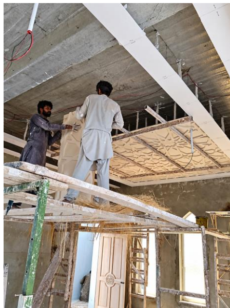
World Federation Alizai Masjid project | Craftsmen installing decorative ceiling components
