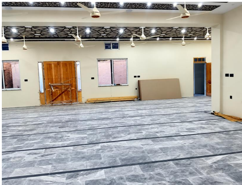
World Federation Alizai Masjid project | Finished prayer hall and floor pattern
