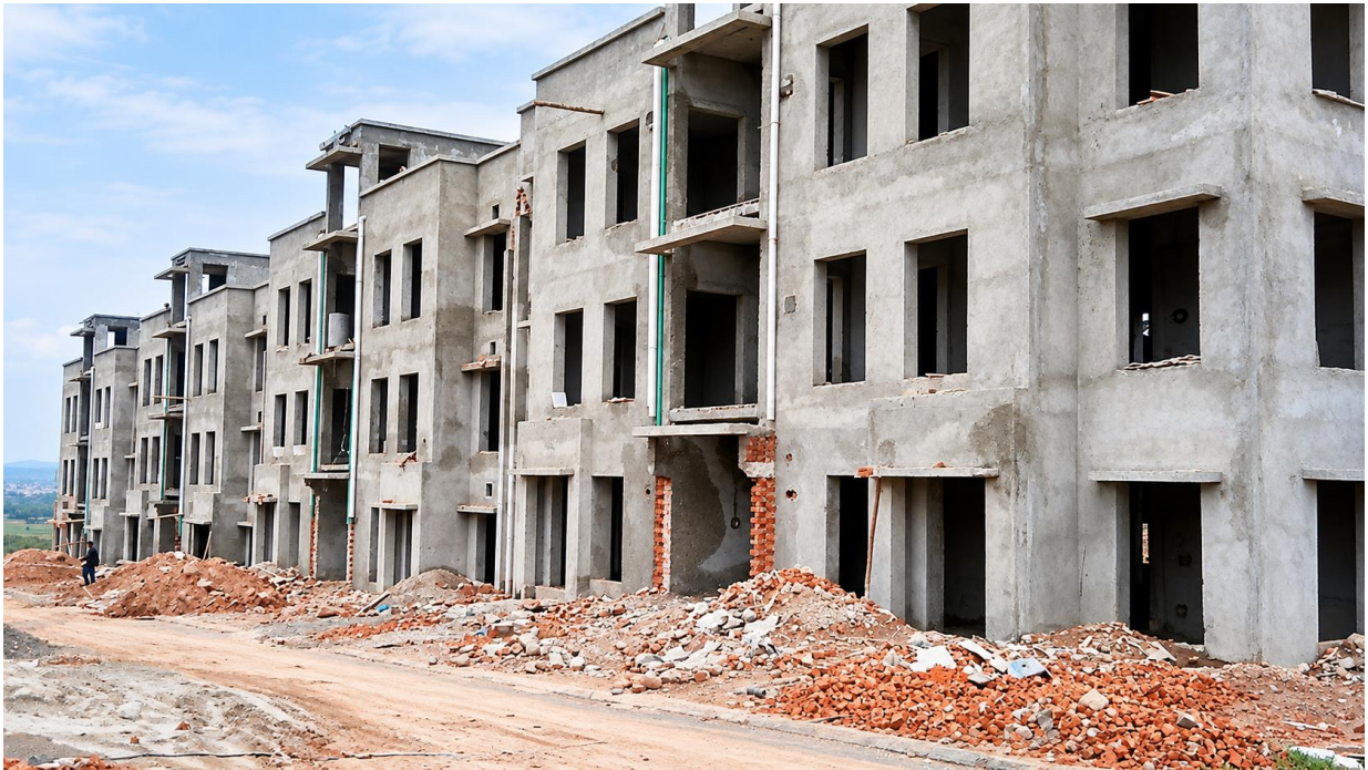
Civil and residential construction portfolio | Multi-storey buildings at plaster-stage completion
