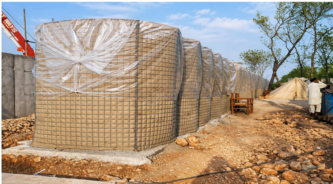
Protective civil works portfolio | HESCO-type barrier installation
