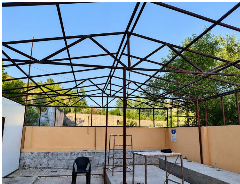
AIMS School and College Islamabad | Steel-frame installation and covered-area development
