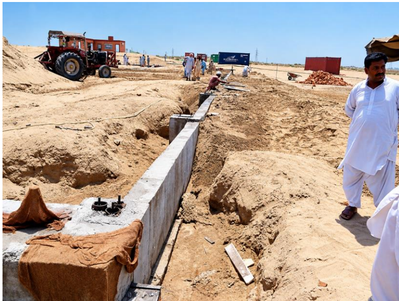
WFP warehouse programme | Foundation alignment across the warehouse site
