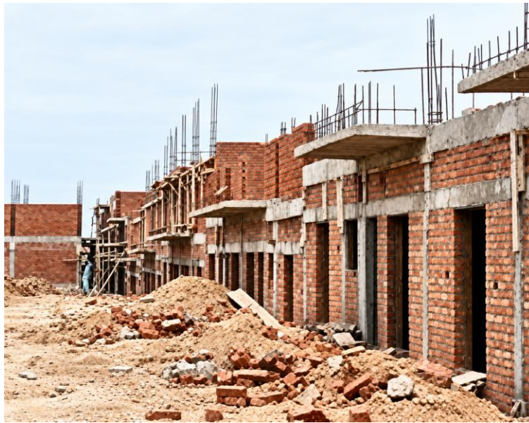
Residential construction portfolio | Reinforced-concrete frame and brickwork
