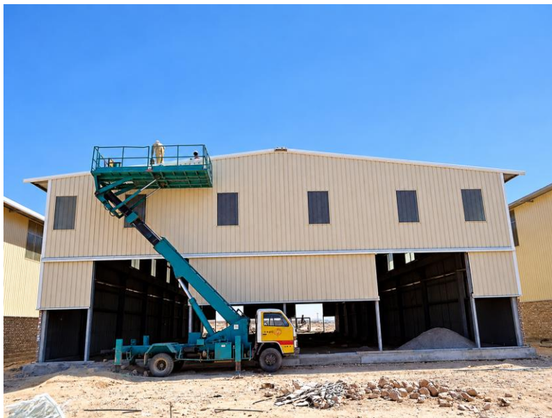
WFP warehouse programme | Warehouse cladding and elevated installation work
