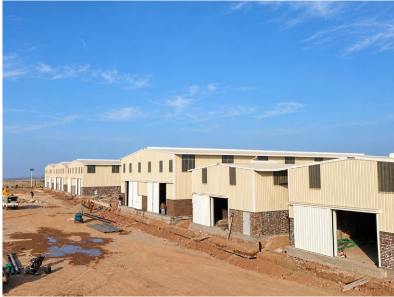
WFP warehouse programme | Completed building envelopes with external works in progress
