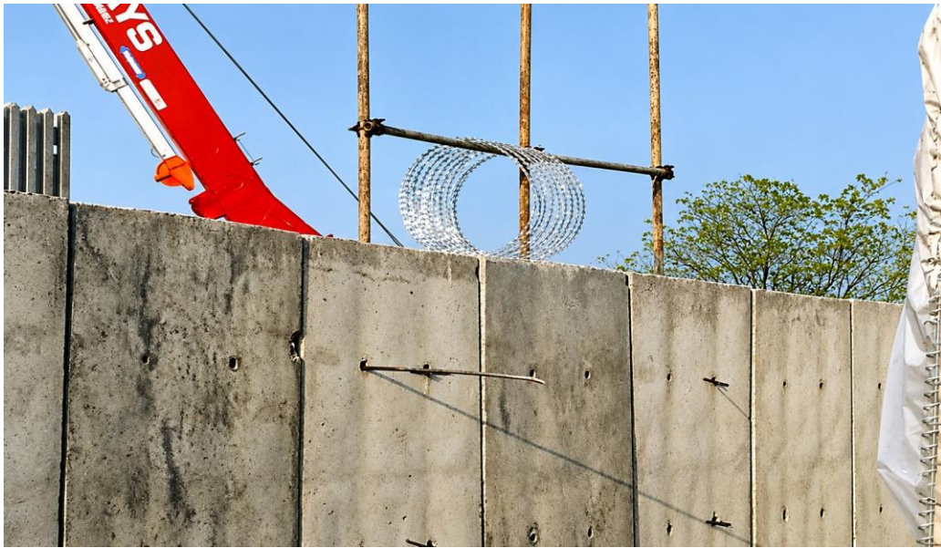
Protective civil works portfolio | Concrete walling and perimeter security
