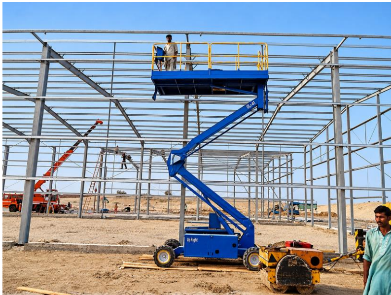
WFP warehouse programme | Elevated access during structural-steel installation
