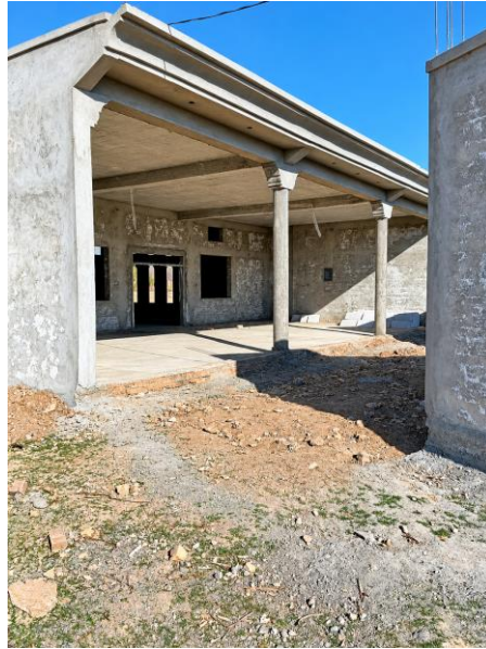
World Federation Alizai Masjid project | Entrance-side view during construction
