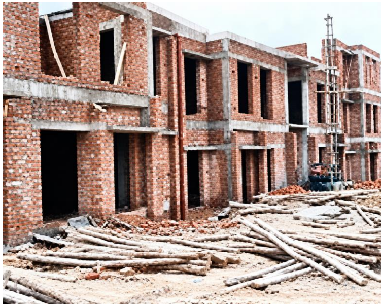
Residential construction portfolio | Brickwork and structural-frame progression
