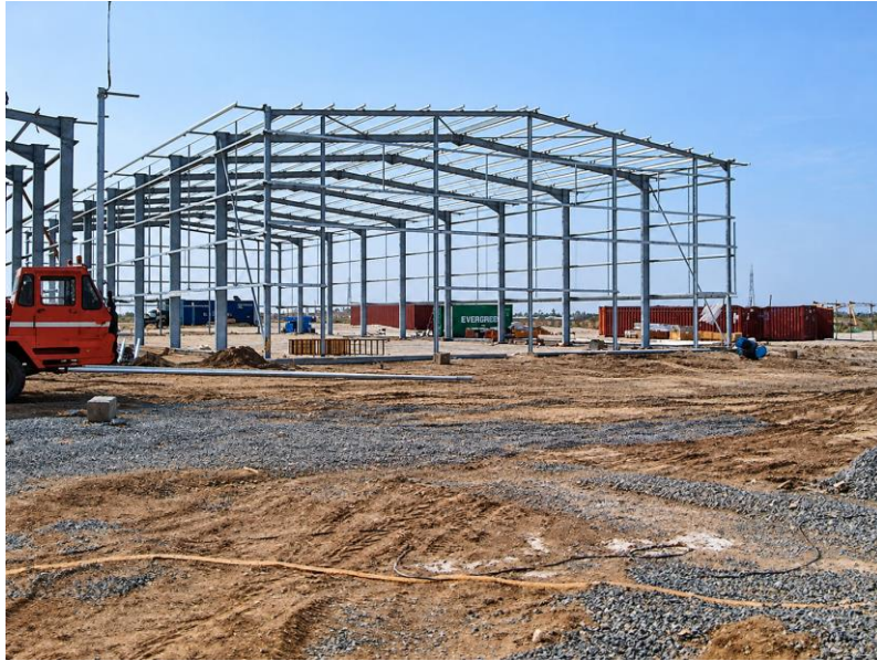
WFP warehouse programme | Warehouse steel frame during assembly
