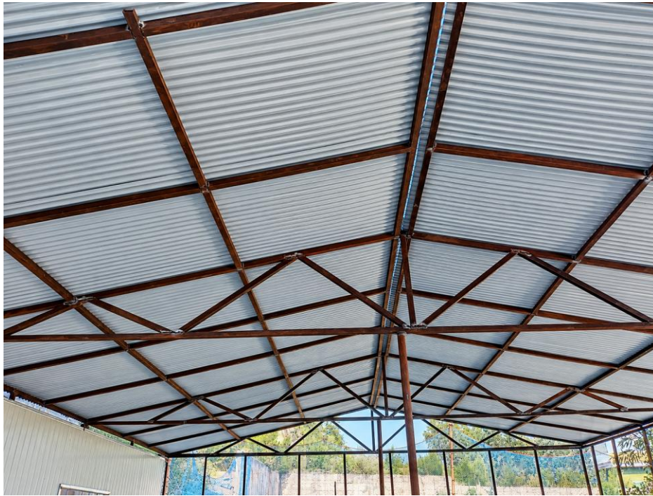
AIMS School and College Islamabad | Completed metal-sheet roofing on fabricated steel trusses
