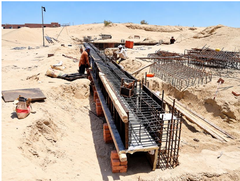
WFP warehouse programme | Reinforcement and formwork during substructure work
