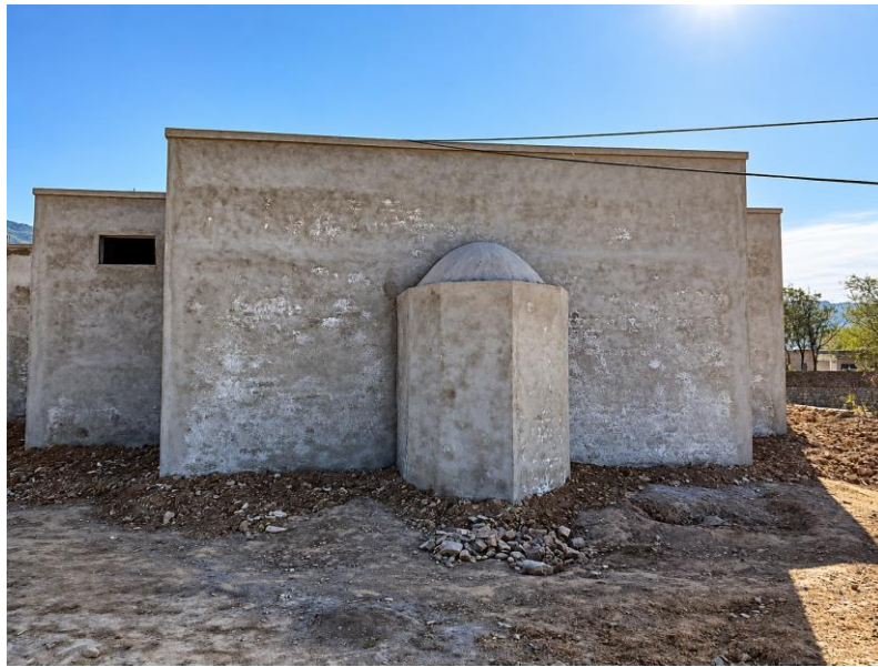
World Federation Alizai Masjid project | External shell after plaster work
