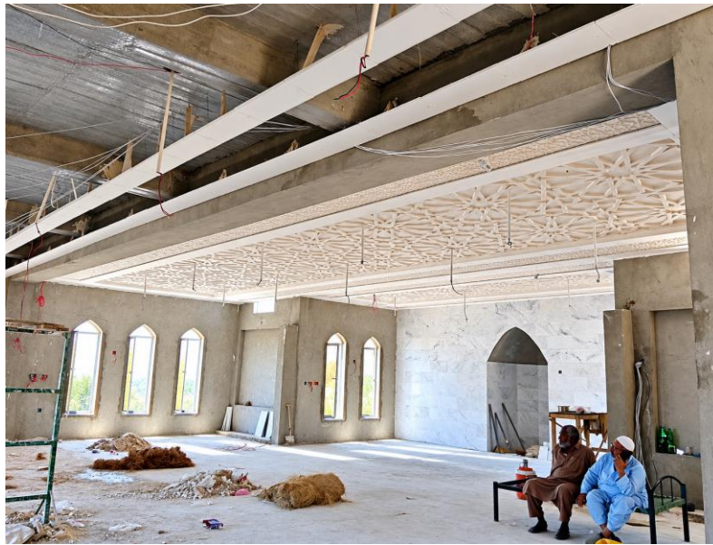
World Federation Alizai Masjid project | Interior works during ceiling installation
