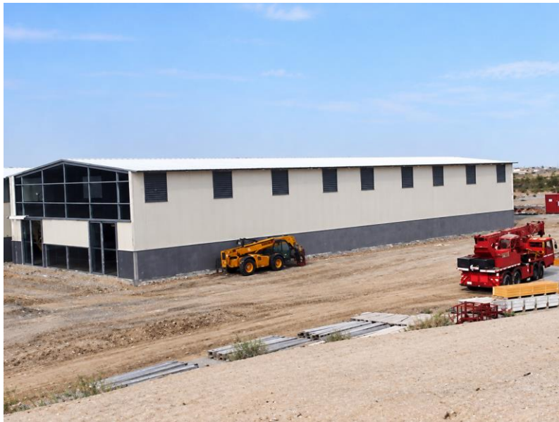
WFP warehouse programme | Clad warehouse building and site equipment
