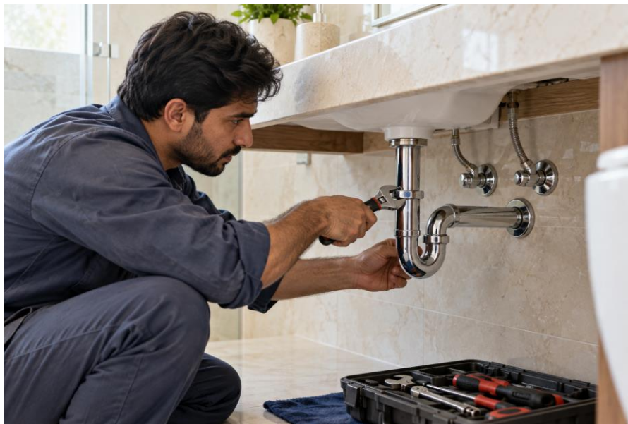
Illustrative service example | Residential plumbing inspection and repair
