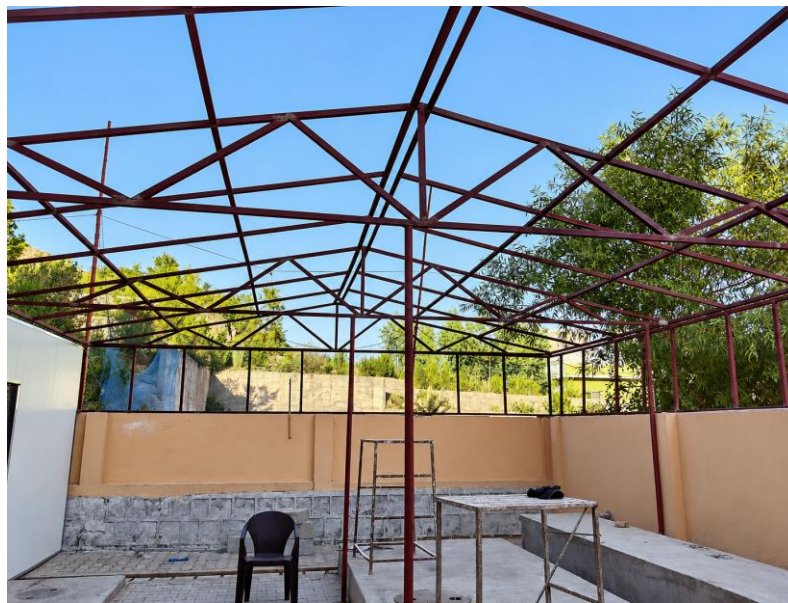
AIMS School and College Islamabad | Pitched steel frame before roof sheeting
