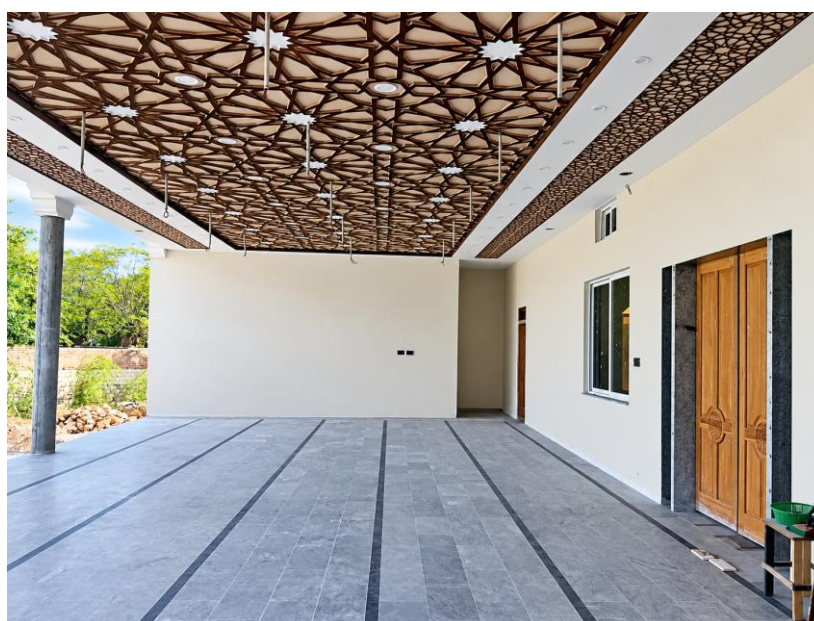
World Federation Alizai Masjid project | Finished entrance portico and geometric ceiling
