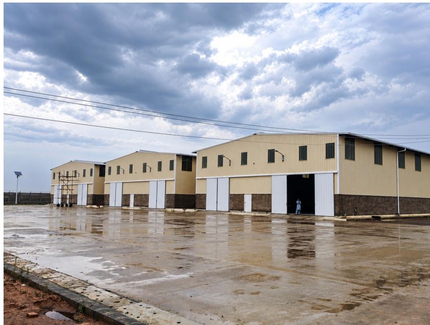
WFP warehouse programme | Finished warehouse exteriors and paved circulation area
