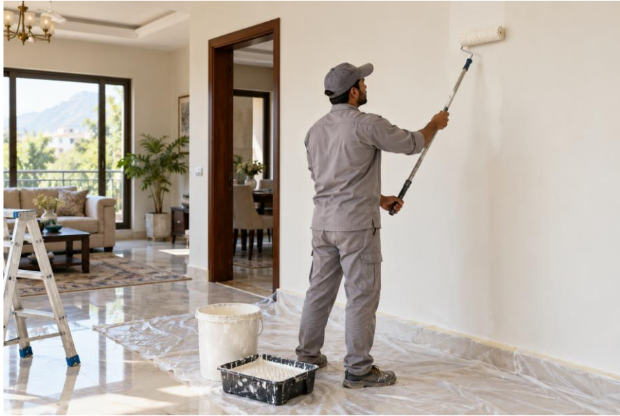
Illustrative service example | Interior repainting and surface maintenance
