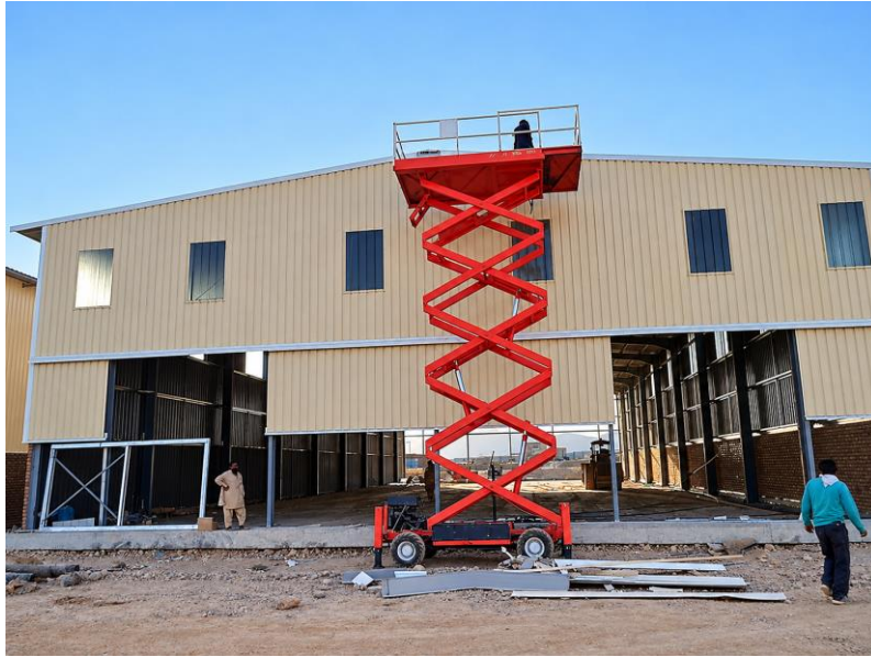
WFP warehouse programme | Facade installation using a mobile lifting platform
