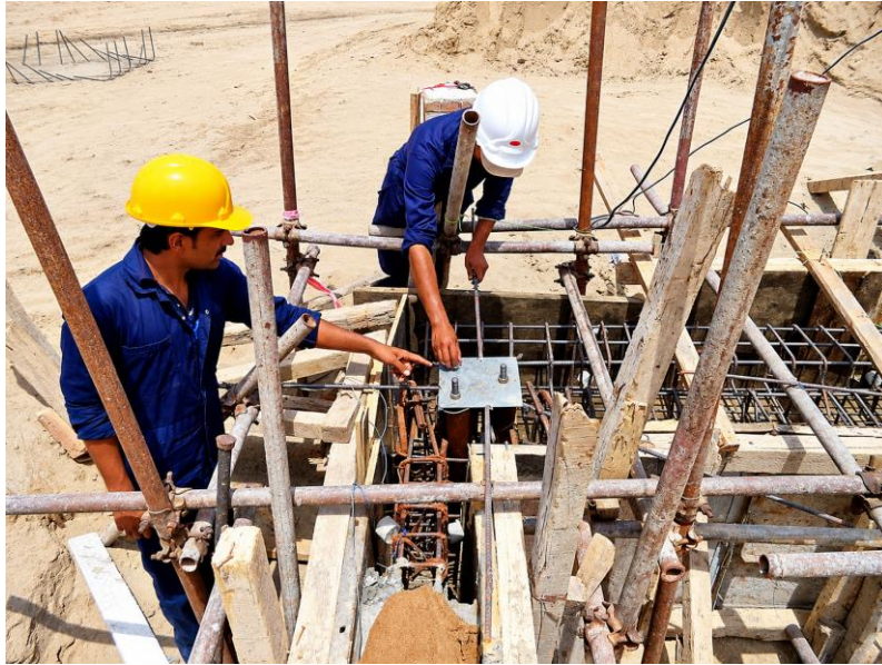
WFP warehouse programme | Foundation and anchor-plate setting with the site team
