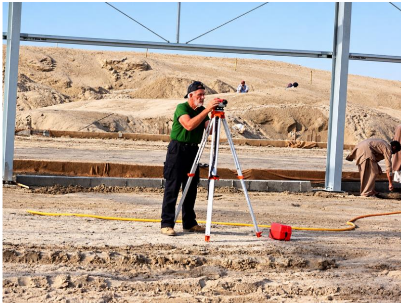
WFP warehouse programme | Survey and level-setting activity during steel erection
