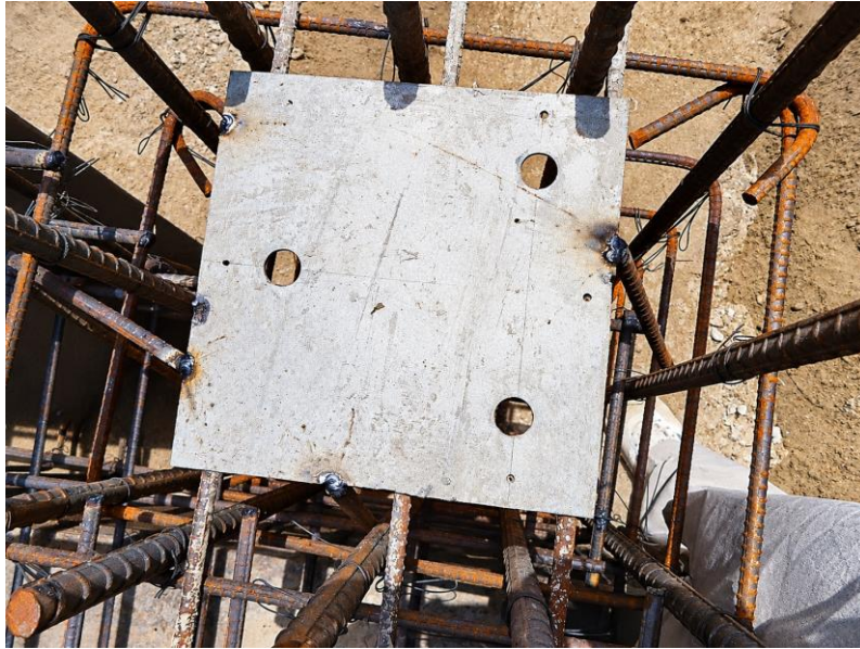
WFP warehouse programme | Anchor-plate and reinforcement detail
