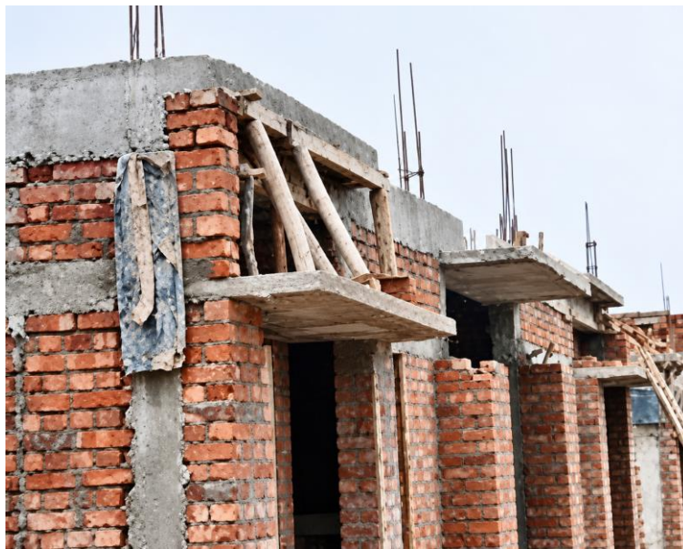
Residential construction portfolio | Slab edges timber supports and masonry
