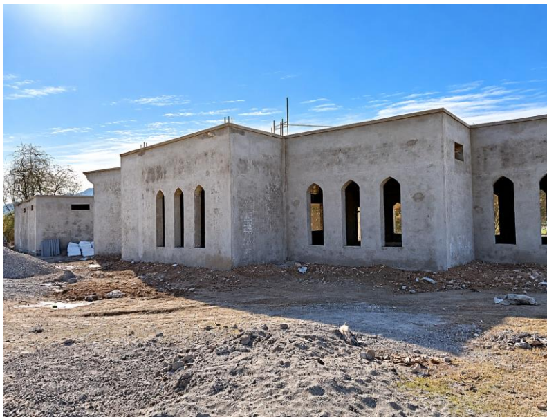
World Federation Alizai Masjid project | Earlier exterior construction stage
