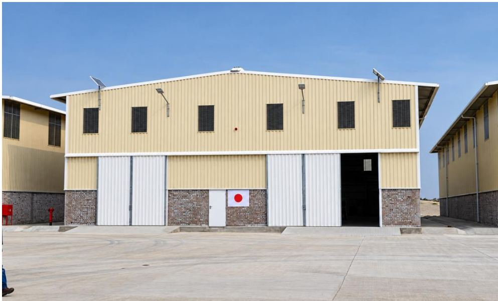
WFP warehouse programme | Finished front elevation and warehouse access openings
