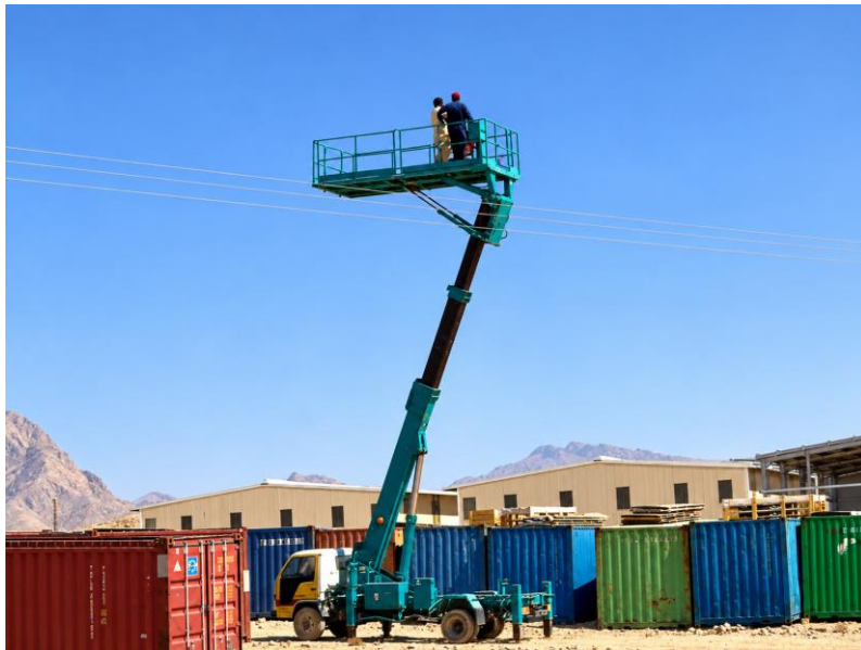
WFP warehouse programme | Elevated site-access equipment supporting erection work
